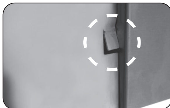
Fig. 25-4 Tab slightly bent in for clearance
